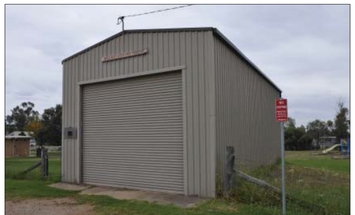
The fire shed that has been positioned in the middle of the Park
