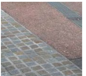
Cobble unit pavers with exposed aggregate
