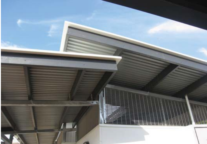
Use of steel for strength and mesh to stop illegal entry while providing high ventilation.
