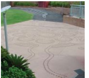
Pressed patterns in coloured concrete
