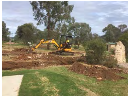
Rehabilitation works at Pensioners Hill
