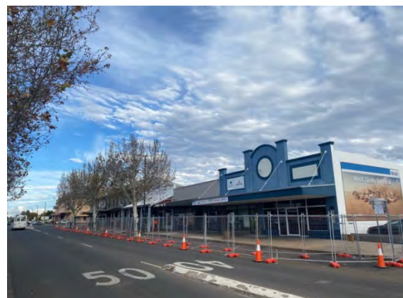
Repaving footpath works in Conadilly Street, between Elgin and Abbott Streets.
