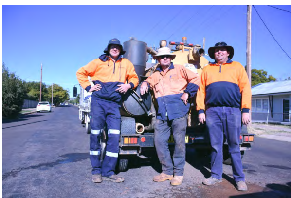
Staff from Council's Water and Sewer Team on the job
