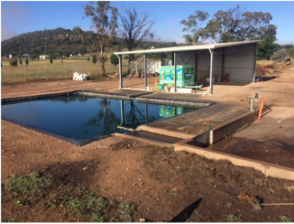
New wash down bay
