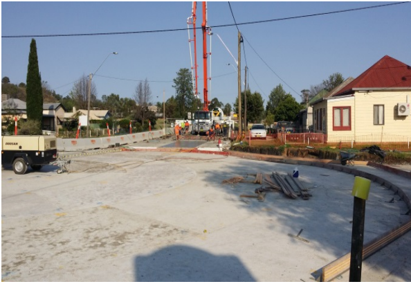
Construction on the Conadilly Street and Warrabungle Street Roundabout
