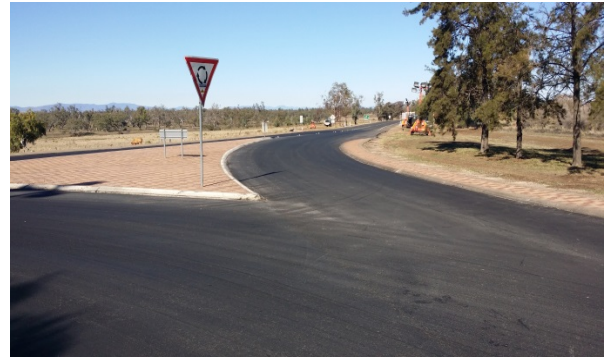
Asphalting the Tamworth/Curlewis roundabout on the Kamilaroi Highway
