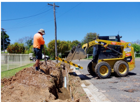
Drainage works being carried out in Wilga Street
