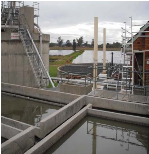
Gunnedah Sewerage Treatment Plant
