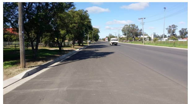
Kerb and gutter works in Bloomfield Street
