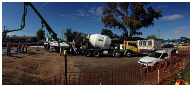
Construction on the Conadilly and Warrabungle Street Roundabout
