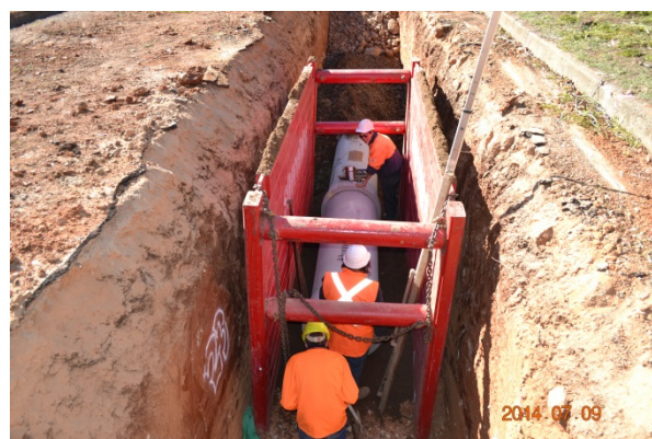
Council staff laying stormwater pipes in Carroll Street.
