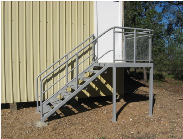
New external stairs at Willala Hall.
