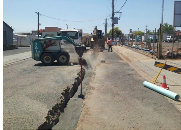
Water main replacement program in Little Barber Street.
